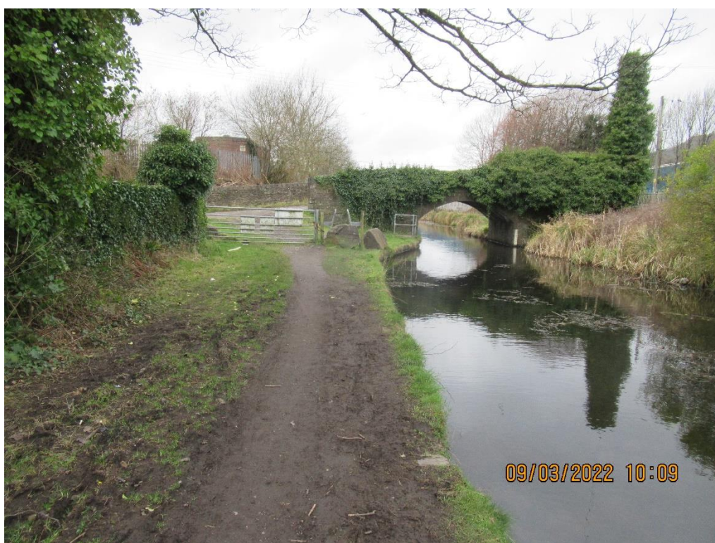
Photo 1: Access bridge over Tennant Canal to Towpath (Bridge South of Abbey reference 11834)
