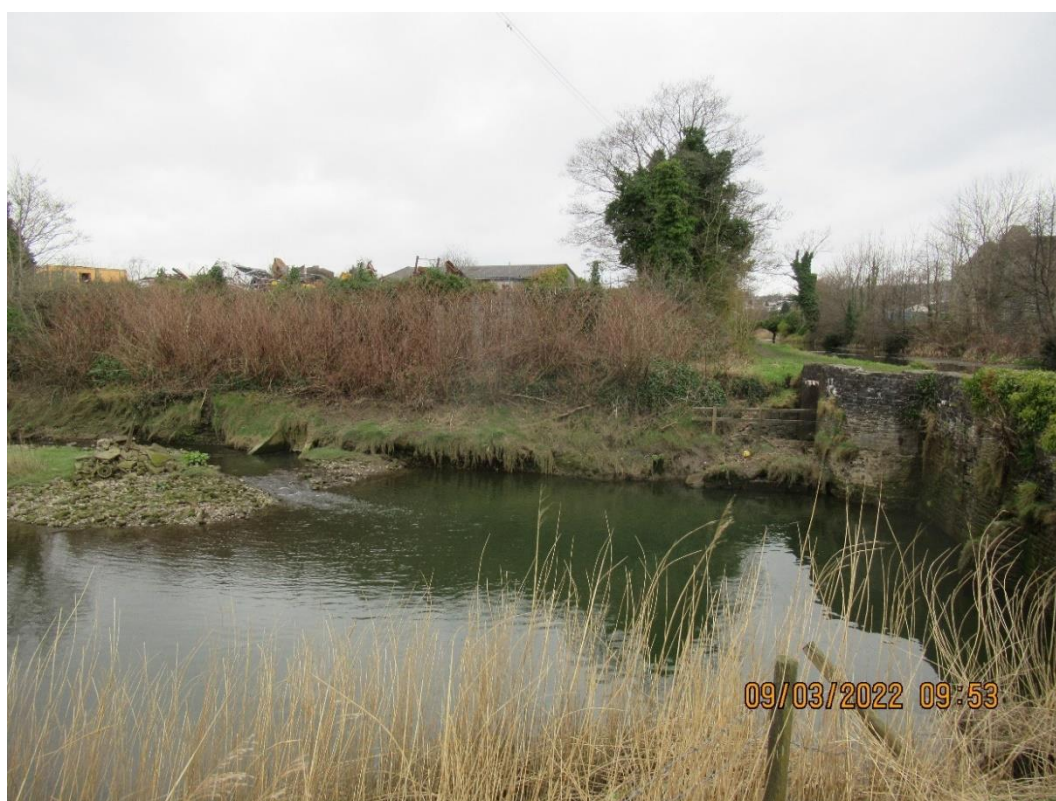
Photo 5: Location of new overflow weir and discharge to River Clydach
