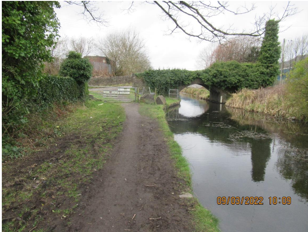
Photo 1: Access bridge over Tennant Canal to Towpath (Bridge South of Abbey reference 11834)
