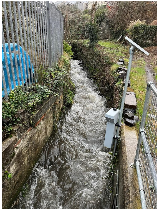
Photograph 8 – Stone walled stream into culvert on Old Road
