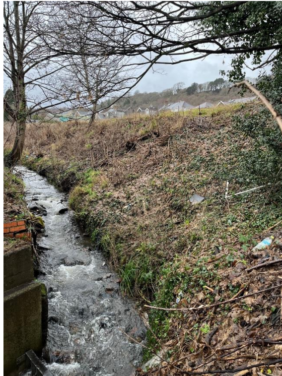
Photograph 1 – Stream into Inlet / Culvert at Caenant Terrace
