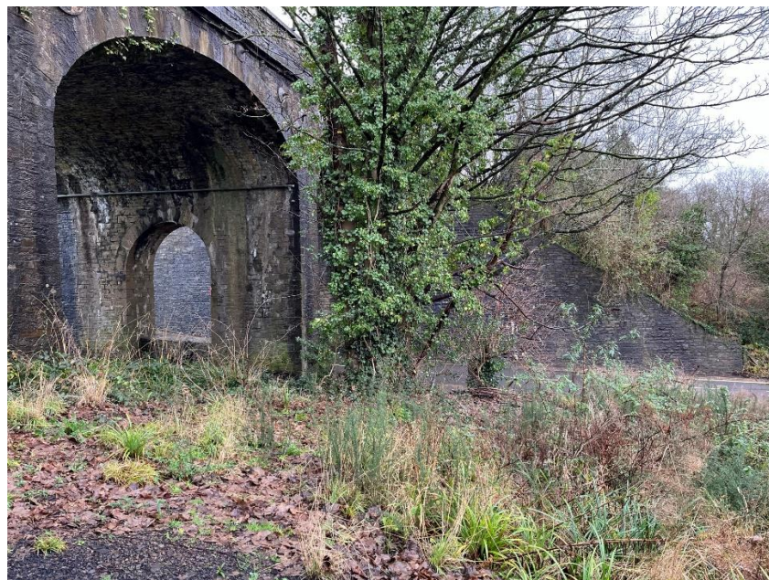
Photograph 4 – Area of scrub adjacent to railway arches on Drummau Road
