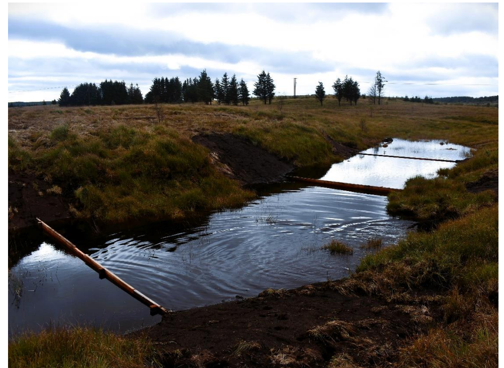
Figure 3: Castell Nos HRA - timber dams in large erosion feature. Image: LPSW
