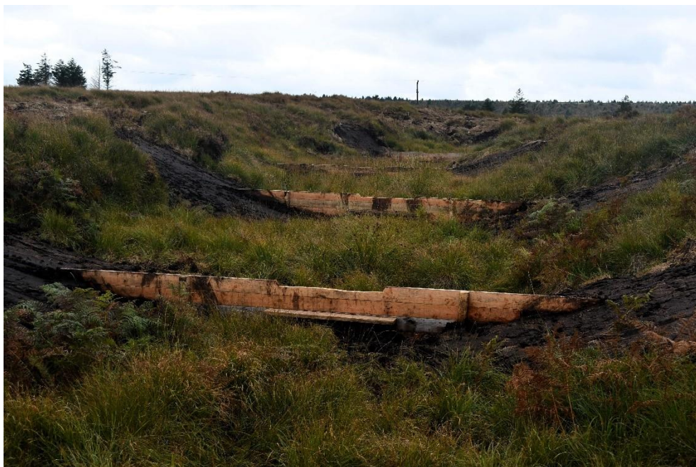
Figure 11: Castell Nos HA - timber dams installed
