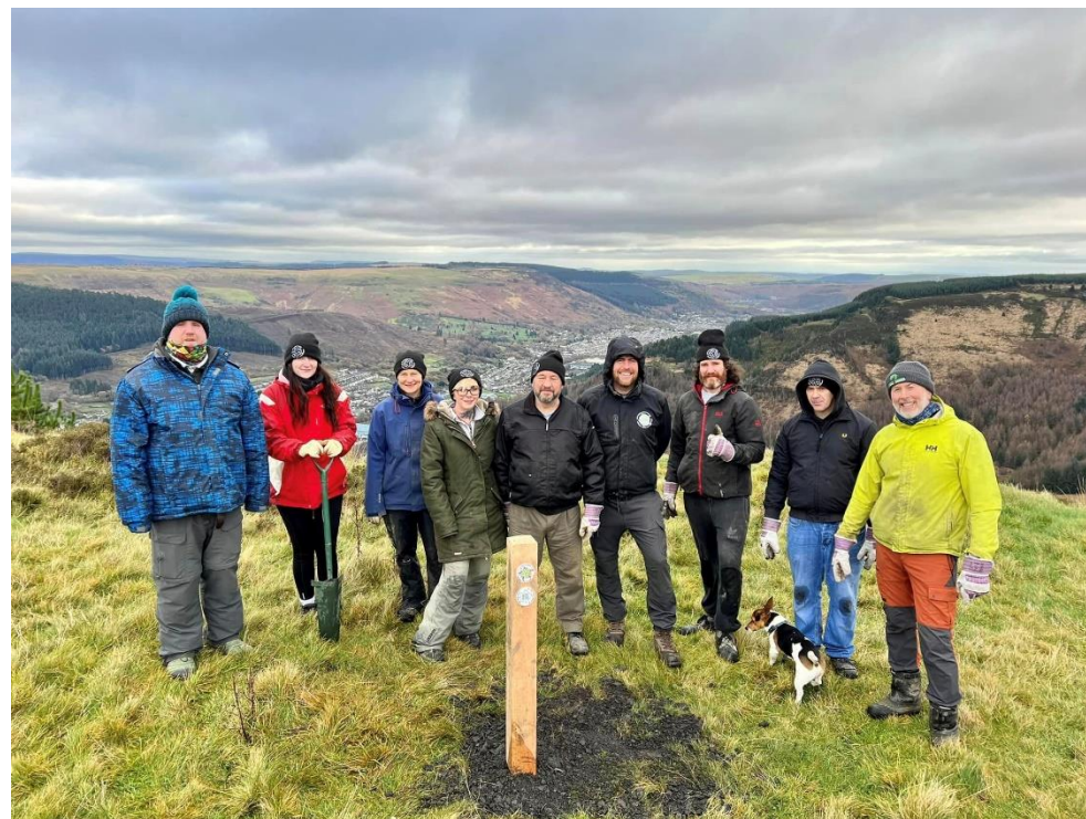
Figure 34: Volunteers install a way marker post at the Cwm Saerbren HRA circular route
