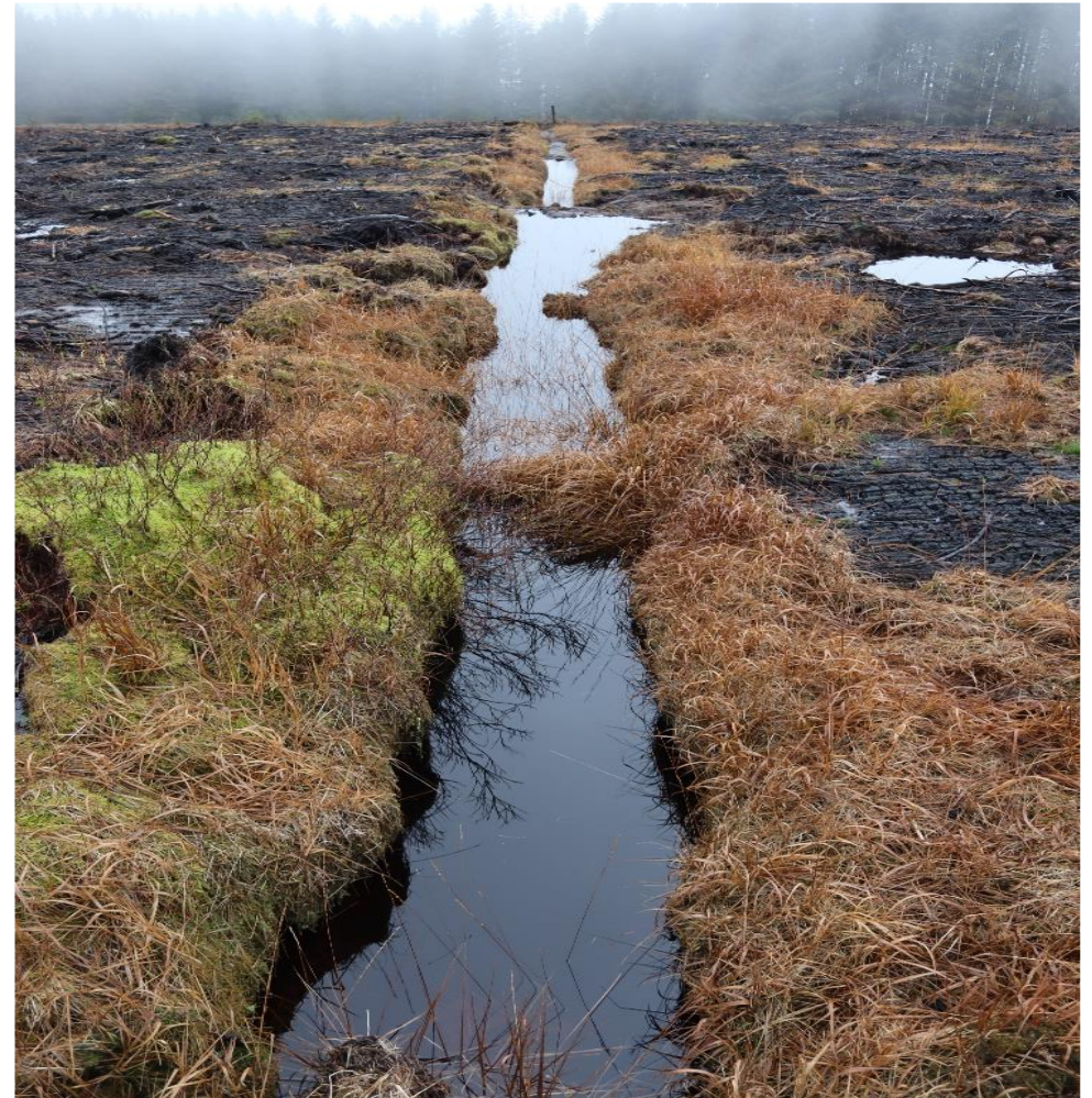
Figure 4: Cregan HRA - large drainage channel blocked with peat dams. Surrounding bare areas had recently been 'ground smoothed'. Image: LPSW
