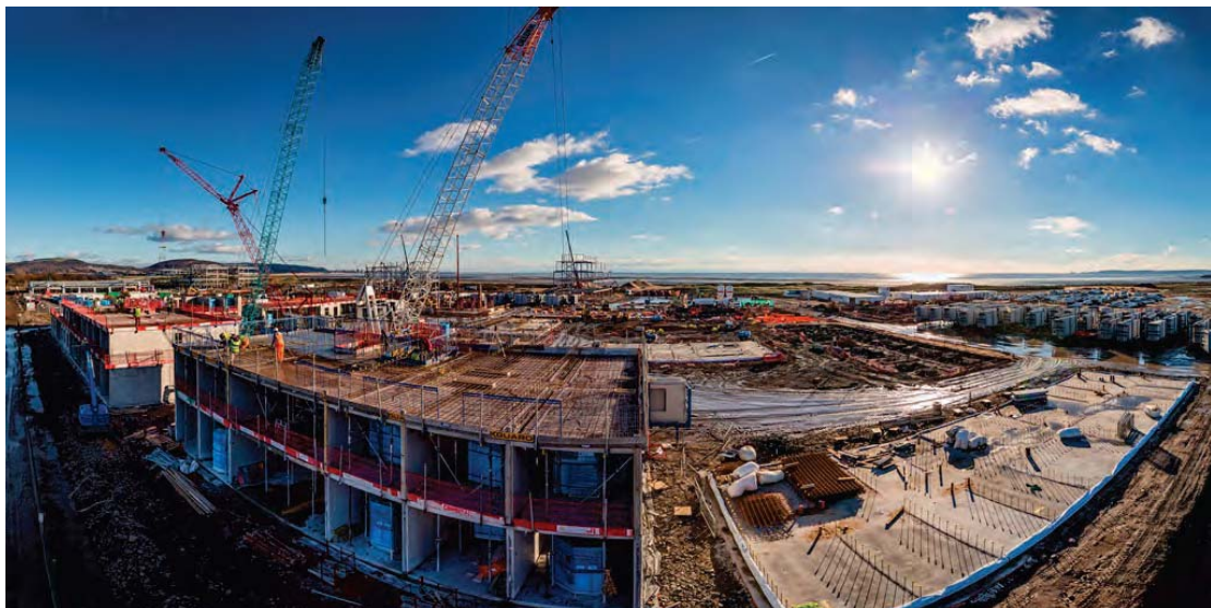
Figure 8. Swansea University Campus under construction
