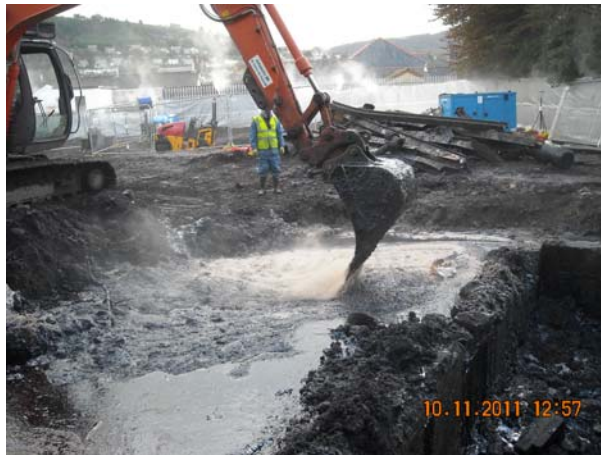
Figure 2. Remediation at Briton Ferry Gas Works
