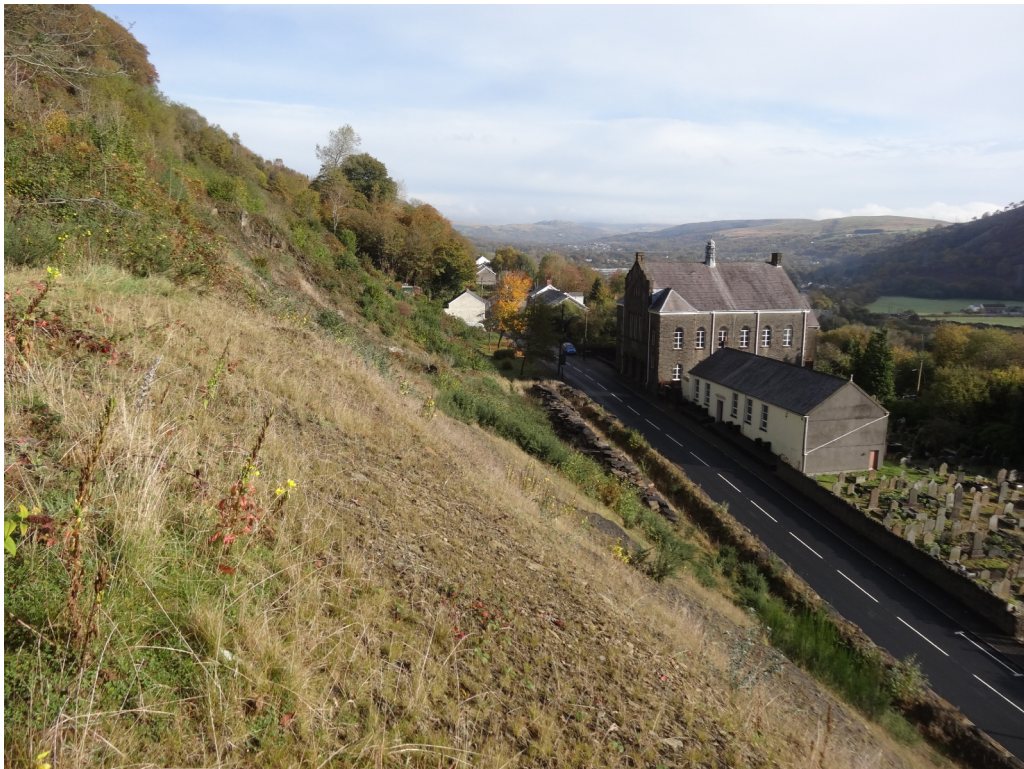
Plate 3: View of 2012 regraded area looking toward Pantteg Chapel
