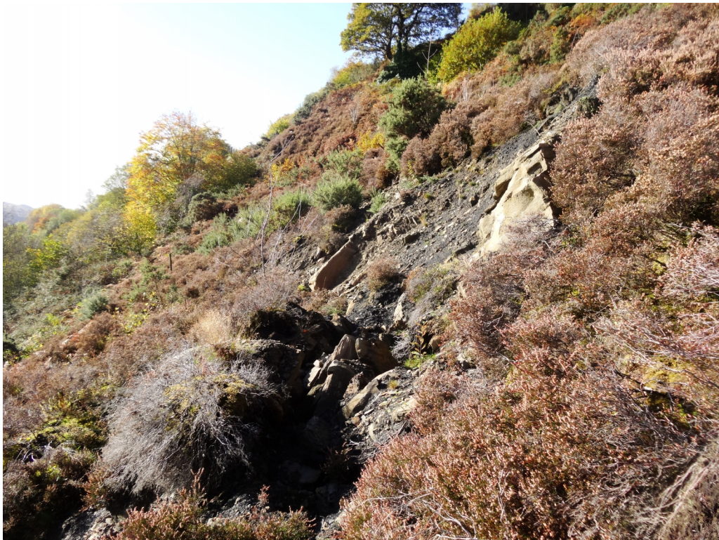
Plate 6: Exposed ground and fissure indicating recent movement.
