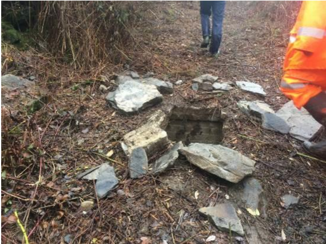
Photograph 17 – Manhole chamber along footpath
