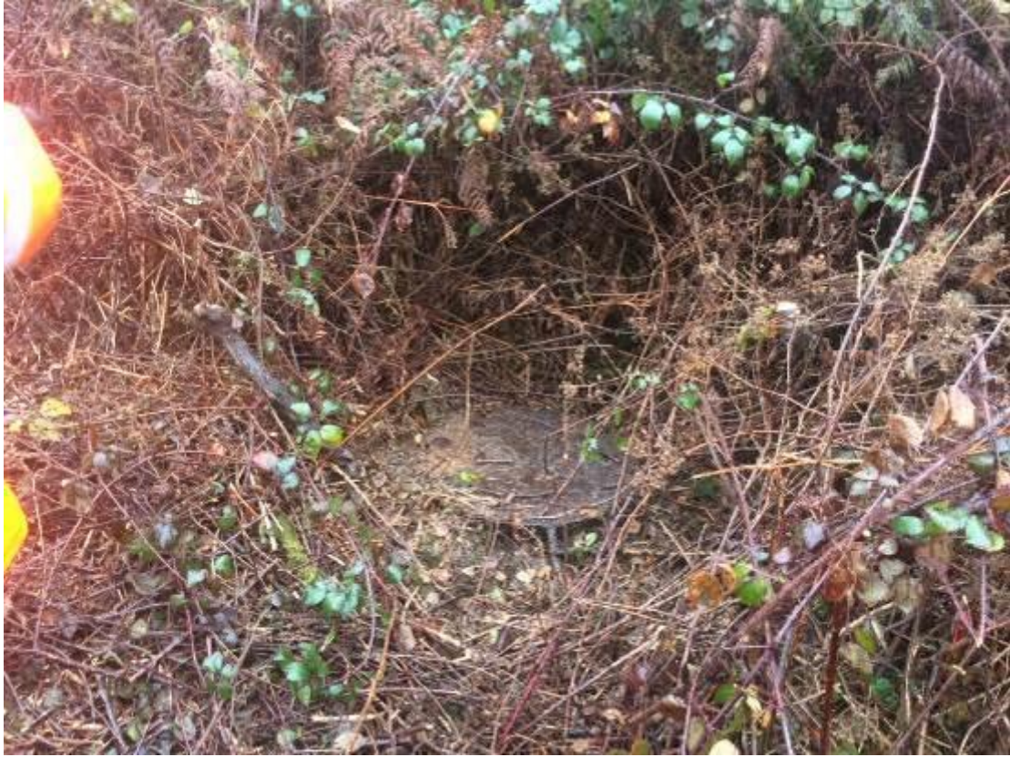
Photograph 13 – Manhole chamber along footpath
