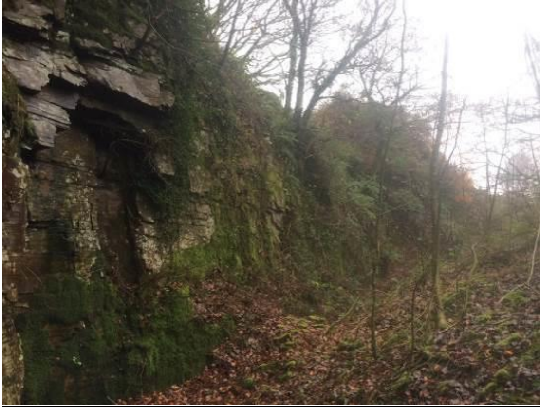
Photograph 5 – Quarry high wall location
