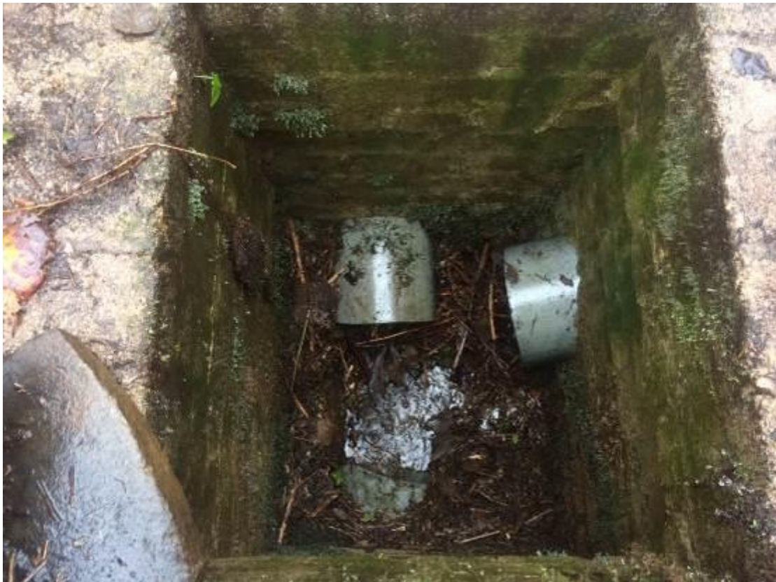
Photograph 14 – Internal view of manhole chamber
