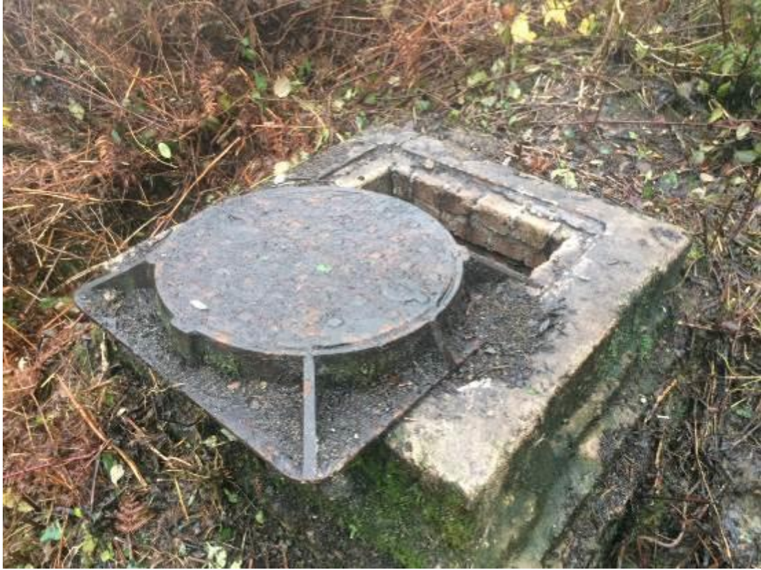
Photograph 15 – Manhole chamber along footpath
