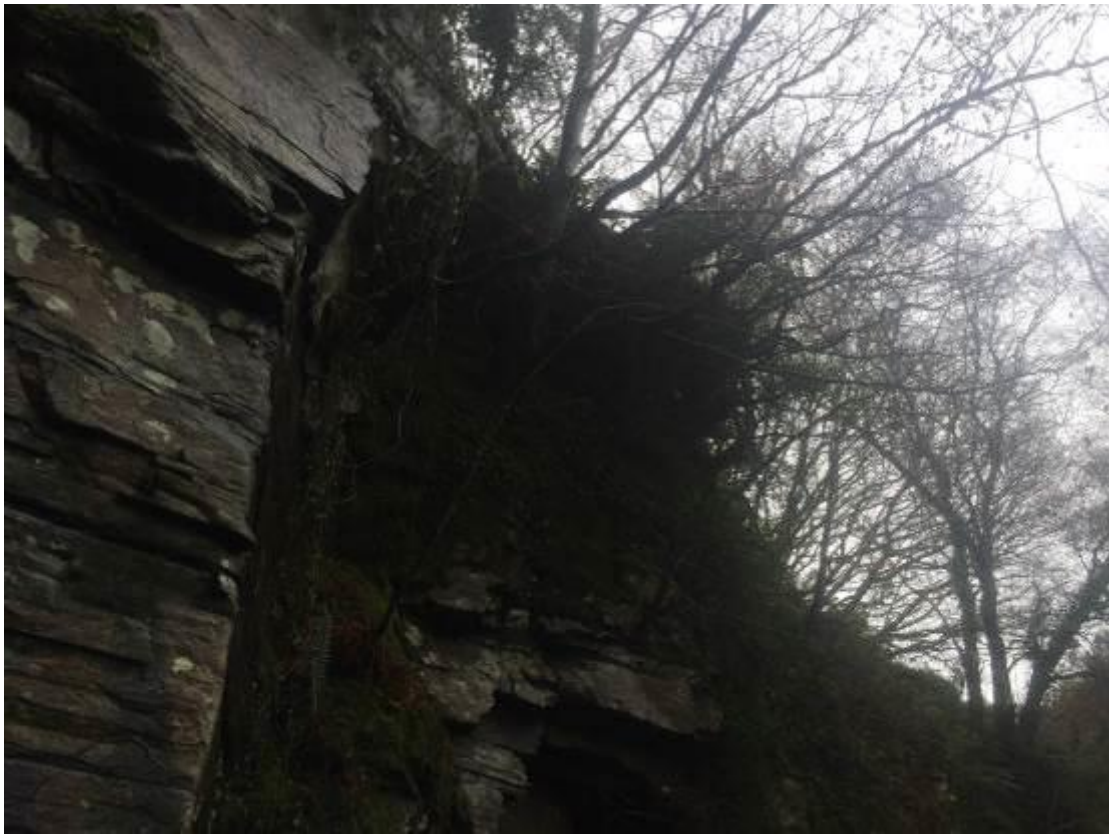
Photograph 6 – Quarry high wall showing overhanging block and trees
