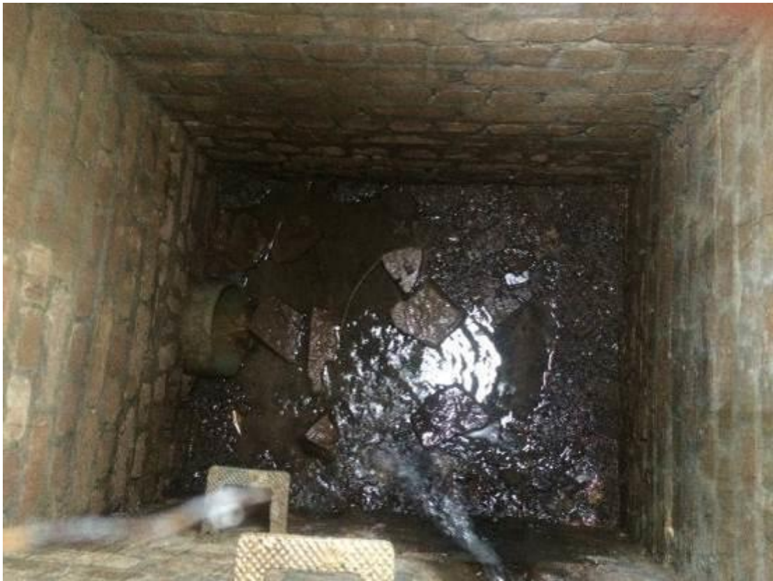
Photograph 16 – Internal view of manhole chamber
