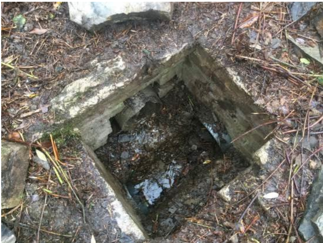
Photograph 18 – Internal view of manhole chamber
