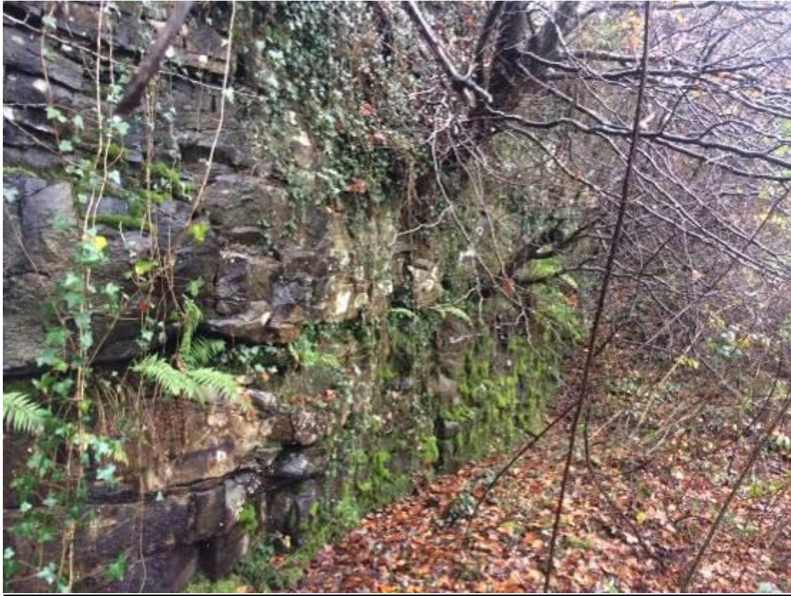
Photograph 1 – Quarry high wall location
