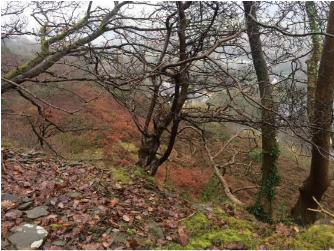
Photograph 12 – Quarry waste toe at crest of cliff
